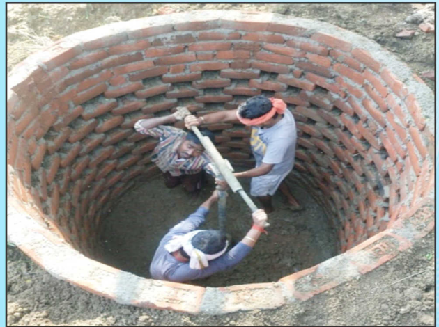
A water recharge pit being dug at Dhaka block (E Ch)
