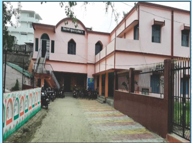
District Central Library, Gopalganj
