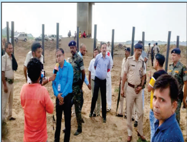
Obstacles embedded on River Bed to curb illegal Movements
